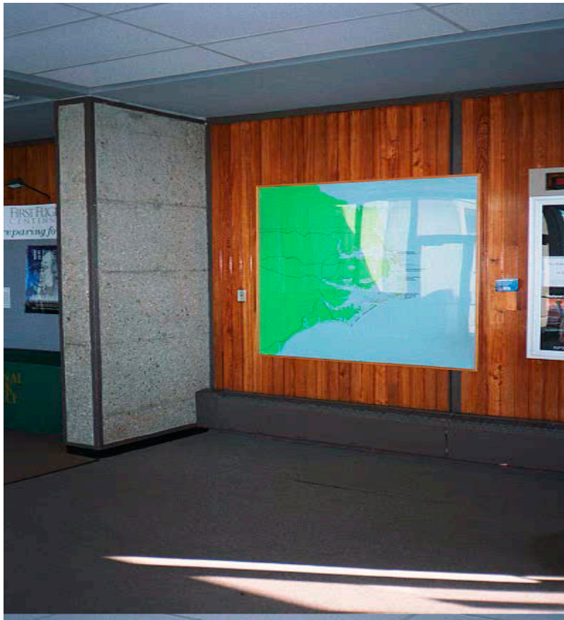
Fig. 5 Lobby of Wright Brothers National Memorial Visitor Center, East Wall, Showing Original Cypress Board Wall and Concrete Column, (2000).
