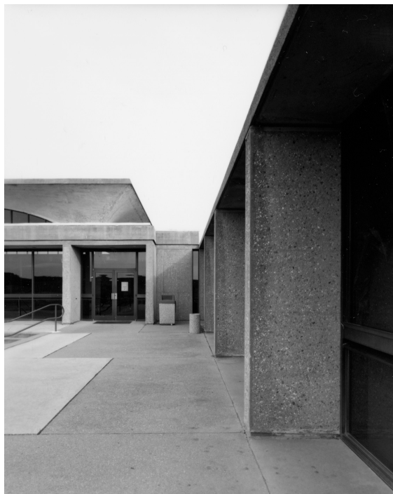
Figure 20 Above, view of concrete paving of Ceremonial Terrace, showing original exposed-large-aggregate panels to right, and the brush finish of modern repairs at left (National Park Service, 2000)
