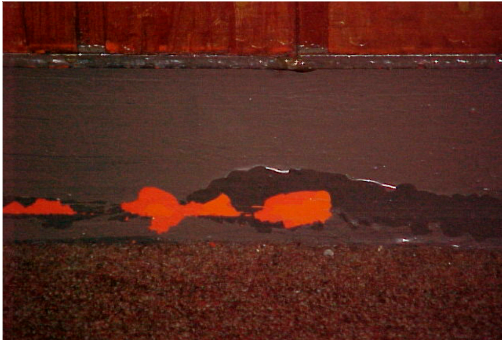
Fig. 8 Detail of Metal Baseboard Trim in Assembly Room of Wright Brothers National Memorial Visitor Center. Note Original Orange Finish, and Later Red-Orange, Dark Brown and Brown-Colored Finishes, (2000).
