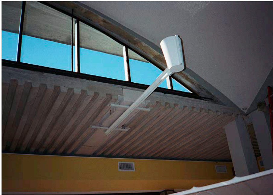
Fig. 10 Original Lamp, Mounting Bracket and Metal Conduit Box Located Beneath the Concrete Soffit of the Assembly Room, Wright Brothers National Memorial Visitor Center, (2000).
