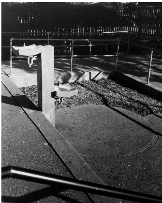
Figure 20 Above, view of concrete paving of Ceremonial Terrace, showing original exposed-large-aggregate panels to right, and the brush finish of modern repairs at left (National Park Service, 2000)
