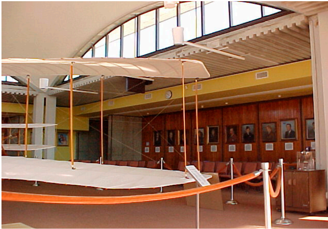
Fig. 9 East Wall of Assembly Room Showing Original Lighting Fixtures, Arched Clerestory Window and Dome Ceiling. Note also the Original Cypress Wall, Enlarged Soffit, and Both the Finished and Unfinished Concrete Columns, (2000).
