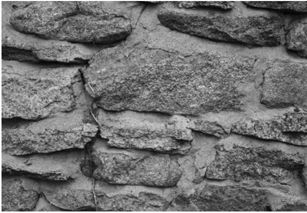
FIGURE 20. View of historic masonry near the southwest corner that has not been repointed. (NPS, 2005)
