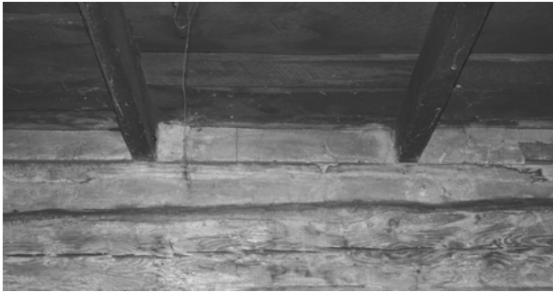
FIGURE 48. View of junction of rafters and sill plate on west side of Room 200. (NPS, 2005)
