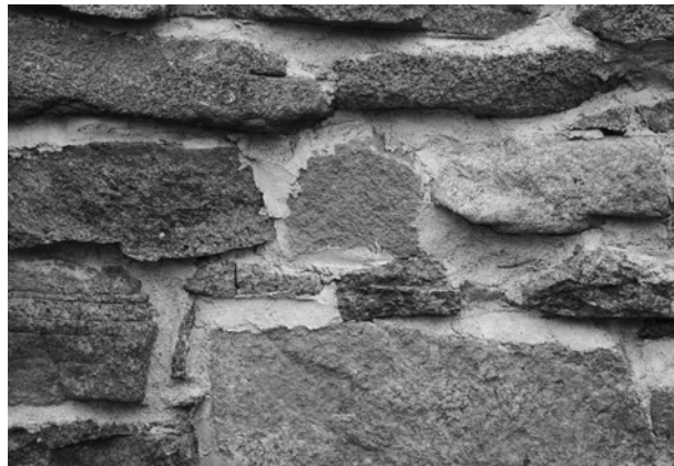
FIGURE 21. View of historic masonry that has been repointed with Portland cement. (NPS, 2005)
