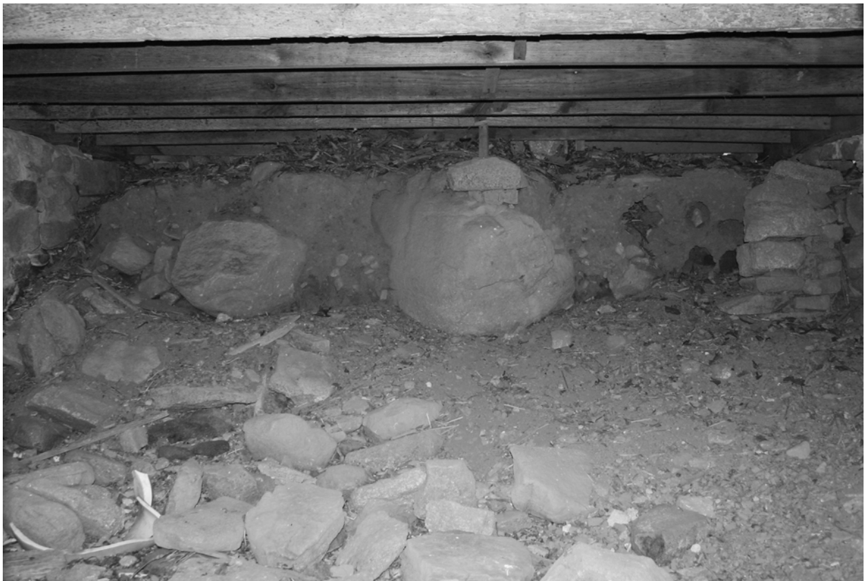
FIGURE 24. View north in cellar, with rocks from collapsed north wall in foreground. (NPS, 2005)
