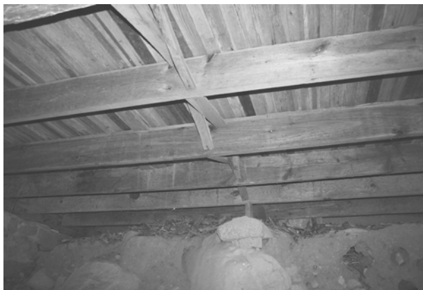
FIGURE 30. View of floor framing in log pen. (NPS, 2005)
