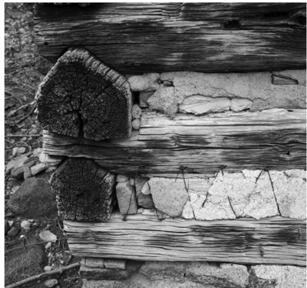
FIGURE 28. View of northwest corner of house, showing typical V-notch corners, all three generations of mortar chinking, and wire lath. (NPS, 2005)
