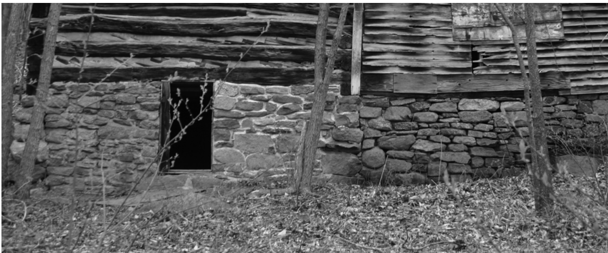
FIGURE 22. View of foundation at south end of house, showing cellar doorway.
