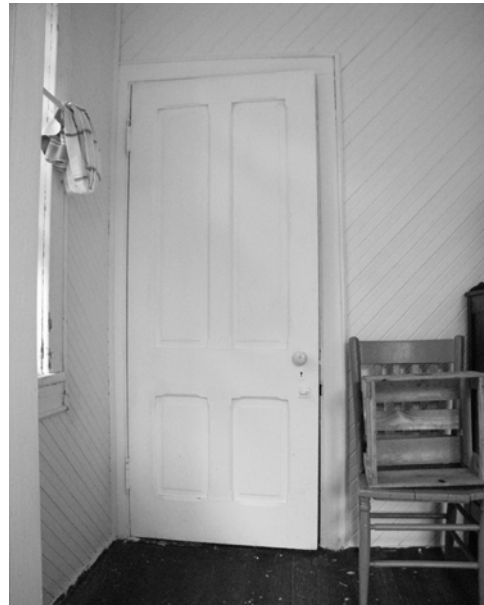
Figure 78 View of original door in Room 202, complete with original mortise lock and porcelain knob. (NPS-SERO-CRS, 2002)
