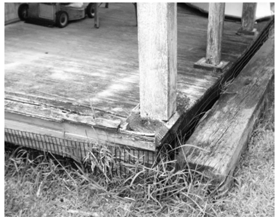
Figure 60 View of northeast corner of front porch, showing corner post seriously destabilized by deterioration of the sills at that location. (NPS-SERO-CRS, 2002)
