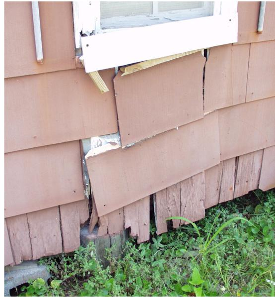
**Figure 24** View of damaged siding on northeast side of house, the result of major sill damage in this location. Original board siding is exposed across bottom of wall. (NPS-SERO-CRS, 2002)
