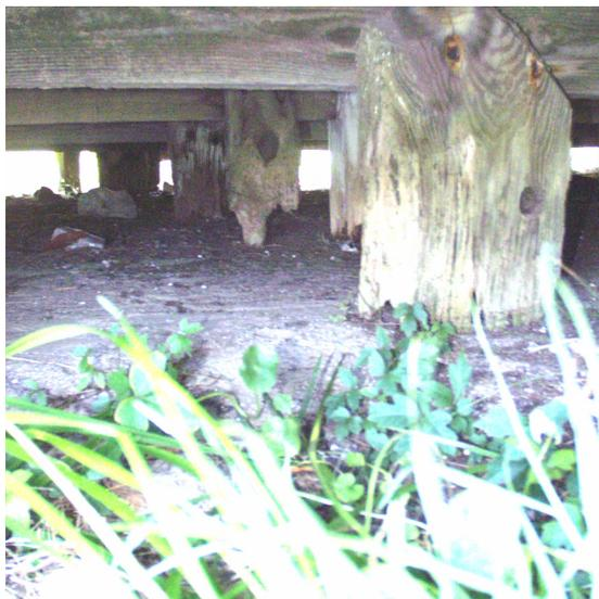
**Figure 20** View of rotted wooden piers that formerly supported floor joists at mid-span. (NPS-SERO-CRS, 2002)
