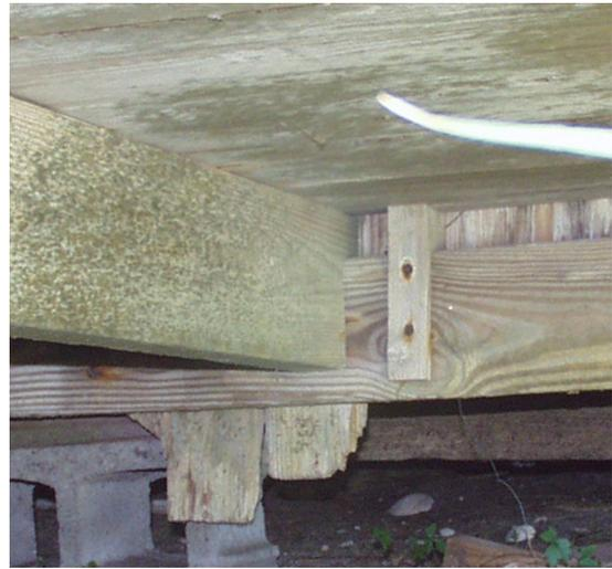
**Figure 21** View of front sill of house and typical joist and stud connections. (NPS-SERO-CRS, 2002)
