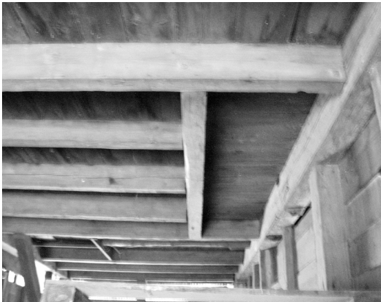
Figure 22 Ceiling in "lint room," showing framed opening for ginned cotton from first or second generation gin at second floor level. (NPS-SERO-CRS, 2001)
