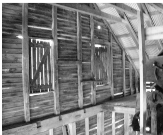
Figure 26 View to southeast showing part of east end of barn; note empty mortises for framing around missing stairway. (NPS-SERO-CRS, 2001)
