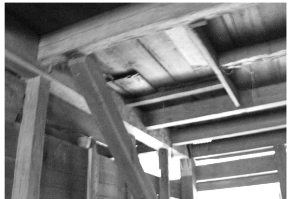
Figure 24 View of framing in lint room ceiling for cotton bale slide which was added along with new hydraulic press around 1900. (NPS-SERO-CRS, 2001)
