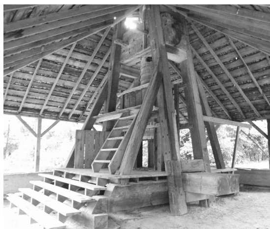
Figure 3 View of interior of Westville press building. Antebellum presses did not always include the surrounding shed, which would have facilitated operation of the press in inclement weather as well as protecting the screw from the elements. (NPS-SERO-CRS, 2001)
