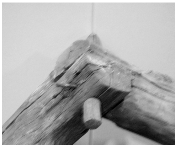
Figure 28 Detail of typical ridge connection in original roof, from partial rafters now in CARI Collection. (NPS-SERO-CRS, 2001)
