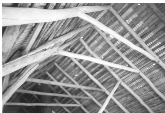
Figure 27 View of original pole-rafter roof in 1995. (NPS-SERO-Architecture, 1995)
