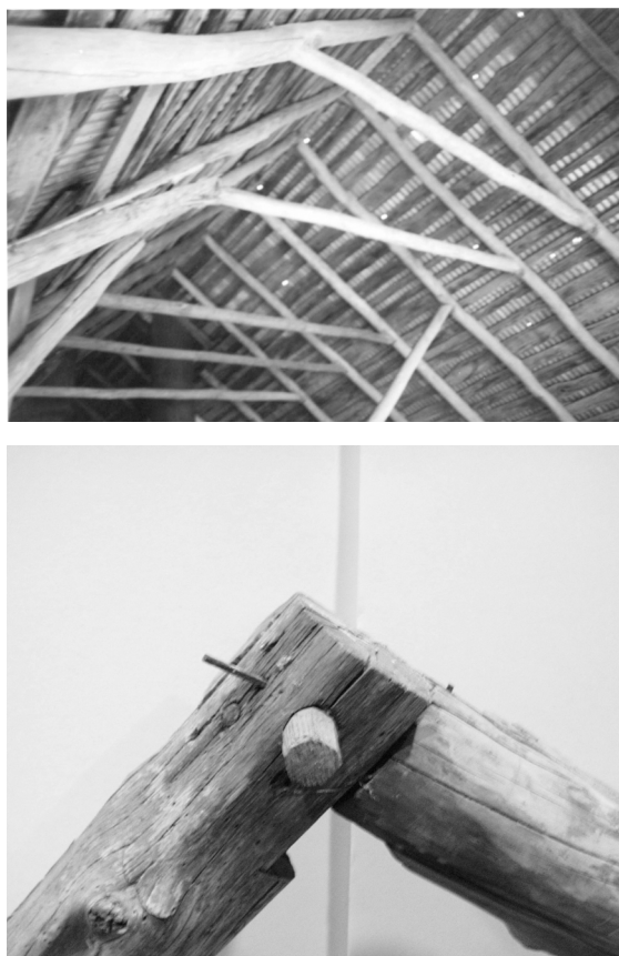
Figure 8 Top, view of original roof prior to its removal in 1995; bottom, detail of salvaged rafters showing lapped and pegged ridge connection. (Upper image, Architectural Division, NPS-SERO, 1994; lower image, NPS-SERO-CRS, 2001)
