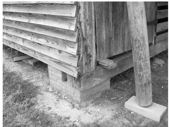
Figure 18 View of northeast corner of barn, showing brick pier rebuilt in 1996. (NPS-SERO-CRS, 2001)
