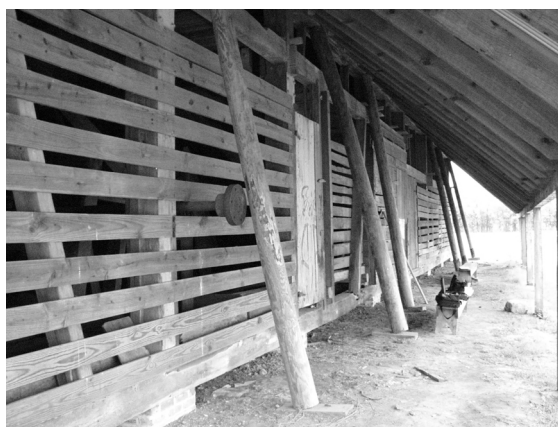
Figure 32 View of north side of building, showing typical open siding. Note that siding near center is attached to the interior face of the studs. (NPS-SERO-CRS, 2001)
