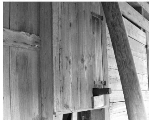
Figure 36 View of window H, which originally had sash but was closed when existing gin machinery was installed c. 1900. (NPS-SERO-CRS, 2001)
