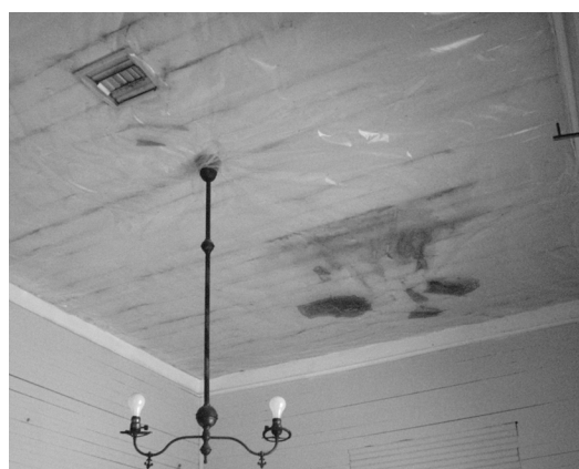
Figure 95 View of water-damaged ceiling in stranger's room. (NPS-SERO-CRS, 2001)
