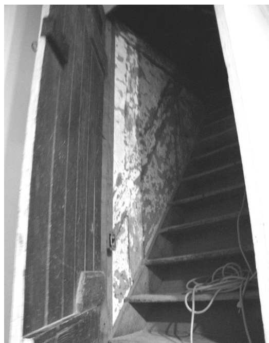
Figure 98 View of attic stairs where one of the early bousillage walls is still visible. (NPS-SERO-CRS, 2001)
