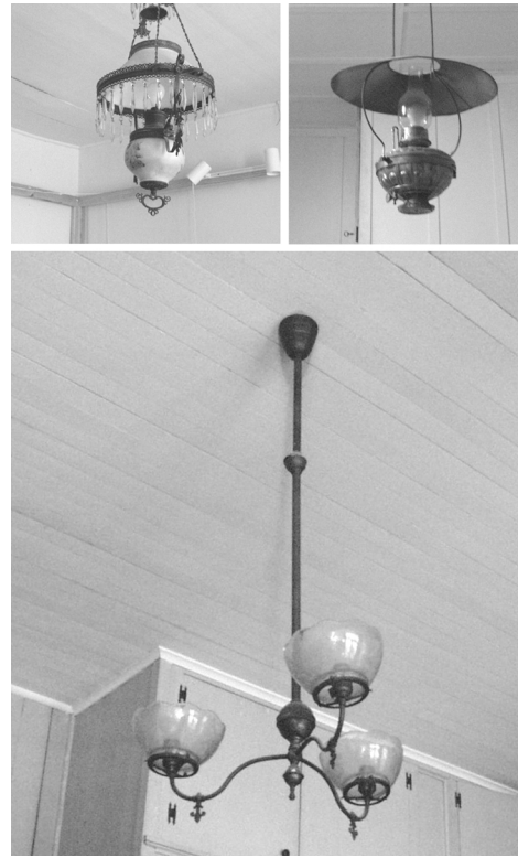
Figure 112 Top, view of nineteenth-century kerosene light fixtures and, below, early twentieth-century gas light fixtures, all of which were converted to electricity in the late 1930s.
