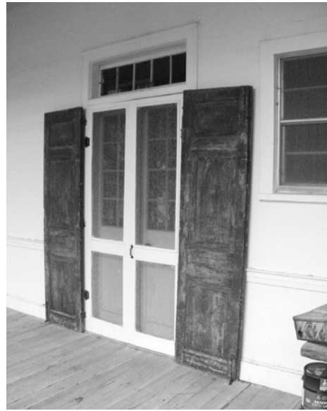
Figure 37 Typical French doors with solid wooden shutters. (NPS-SERO-CRS, 2001)
