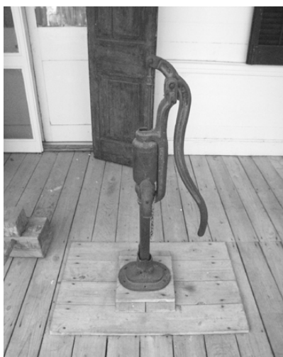
Figure 48 Myers pump on rear gallery, still connected to cistern located below. (NPS-SERO-CRS, 2001)
