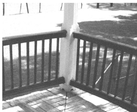
Figure 45 Typical gallery post, balustrades, and flooring. (NPS-SERO-CRS, 2001)
