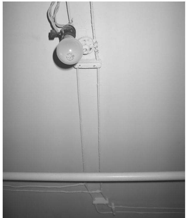
FIGURE 69. View of a portion of the knob-and-tube wiring system, which is no longer active. (T. Jones, NPS, 2004)
