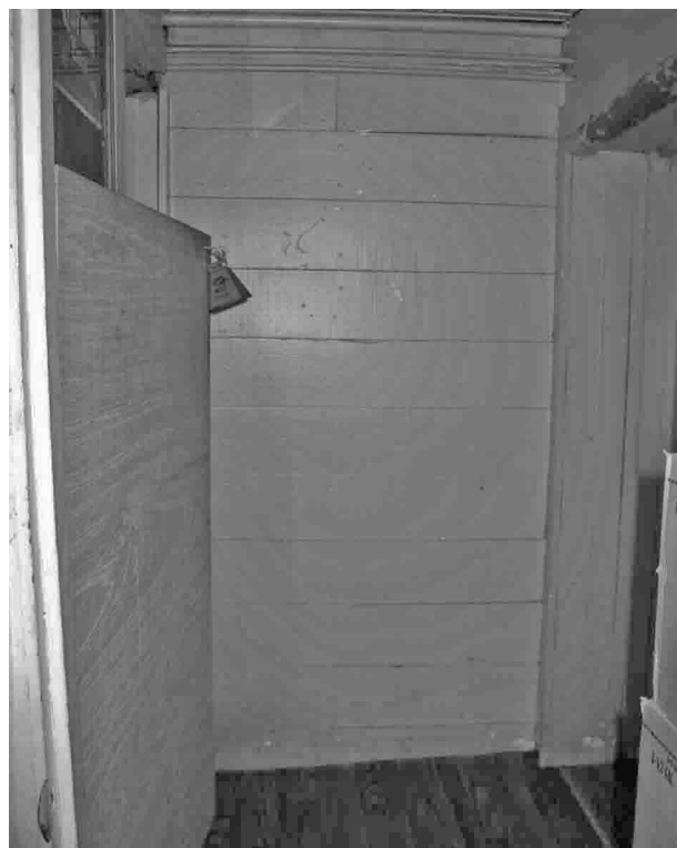
FIGURE 42. View of board walls in hall, typical of original wall finishes in the small pen.
