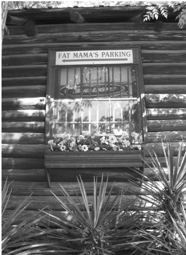
FIGURE 36. View of Window A, which is an original opening that has been altered to fit modern sash.
