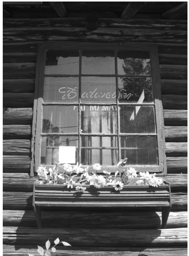
FIGURE 35. View of Window C, the only relatively unaltered original window in the building.
