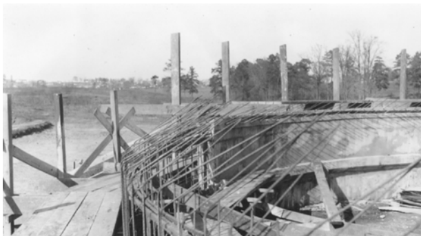
FIGURE 30. View of Earth Lodge, February 2, 1937, with north half of wall complete and rebar in place for south half. (Swanson, OCMU Coll.)
