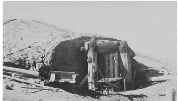
FIGURE 45. View of construction of entrance to Earth Lodge. (OCMU Coll.)
