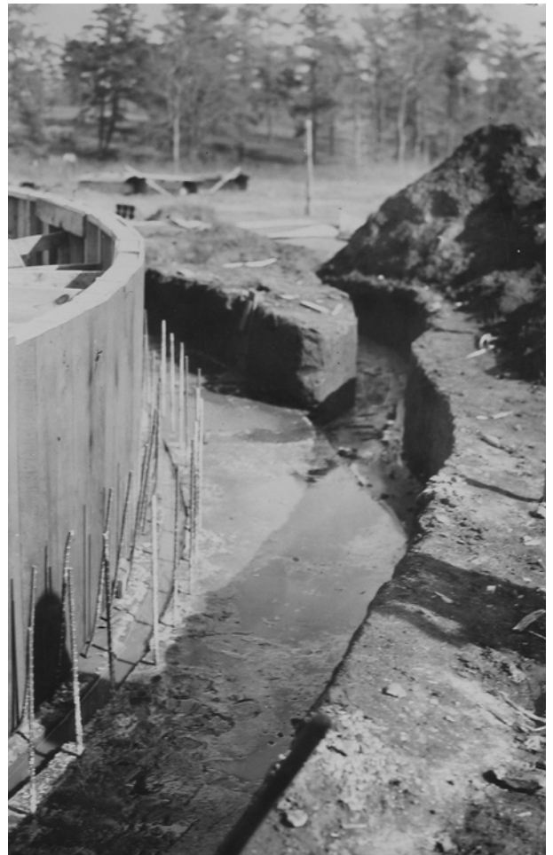
FIGURE 28. View of footings, with one side of the wooden forms and the rebar for the first pour of walls in place. (Swanson, OCMU Coll.)
