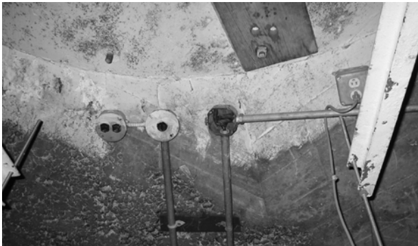
FIGURE 117. View at top of inside of concrete shell, showing remnants of 1937 electrical system and of white paint applied to improve the day-light effect of the original lighting. (NPS-SERO-CR, 2004)
