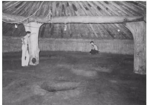
FIGURE 39. View of interior of lodge after removal of protective sand layer but prior to reconstruction of clay walls. (Swanson, OCMU Coll.)
