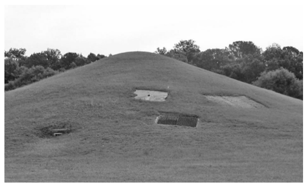
FIGURE 82. View east showing grates and access doors for mechanical pits added in 1975. (NPS-SERO-CR, 2004)
