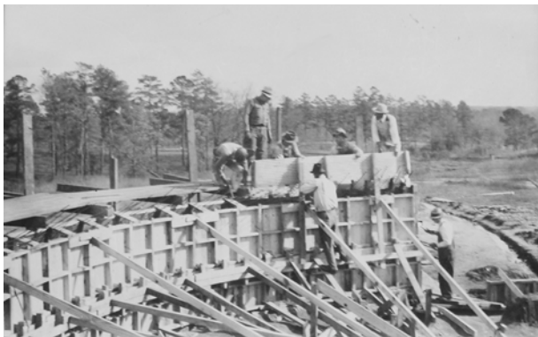
FIGURE 29. Pouring upper portion of north half of concrete wall, January 22, 1937. (Swanson, OCMU Coll.)
