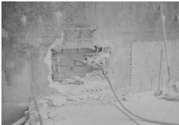
FIGURE 91. View of concrete shell at west end of electrical room showing presumed typical relationship between the concrete wall and the mud-brick wall behind. (Kidd and Associates, 1975))
