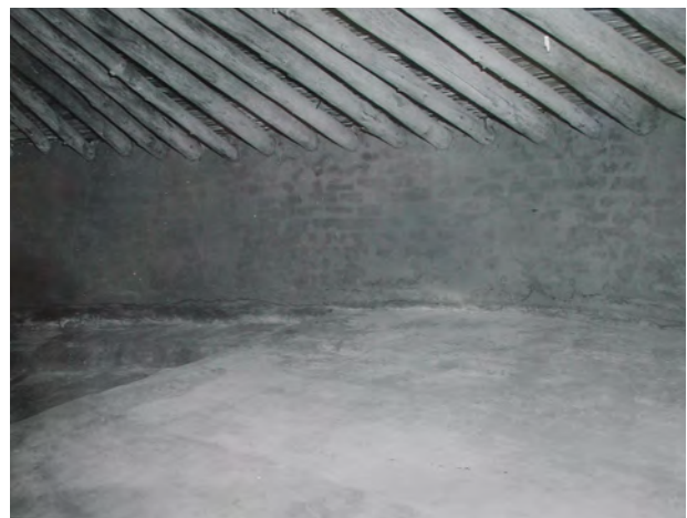
FIGURE 63. View west in Earth Lodge, showing discoloration of reconstructed wall due to uneven moisture penetration, 1965. (OCMU Coll.)
