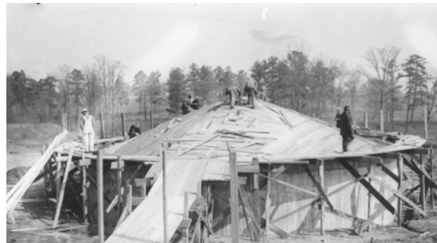
FIGURE 33. View of completed form for roof, March 1, 1937. (Swanson, OCMU Coll.)
