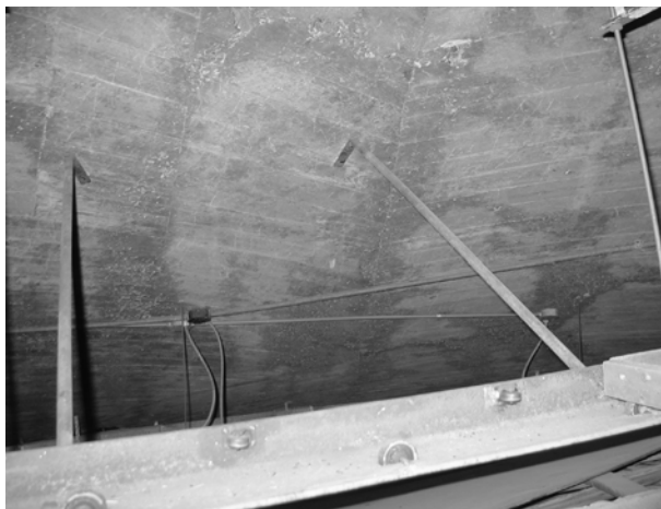
FIGURE 92. View of underside of roof of concrete shell, with imprint of wooden forms clearly visible. (NPS-SERO-CR)
