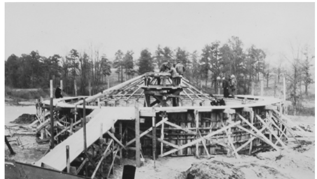
FIGURE 32. View of construction of false work for pouring concrete roof. (OCMU Coll.)
