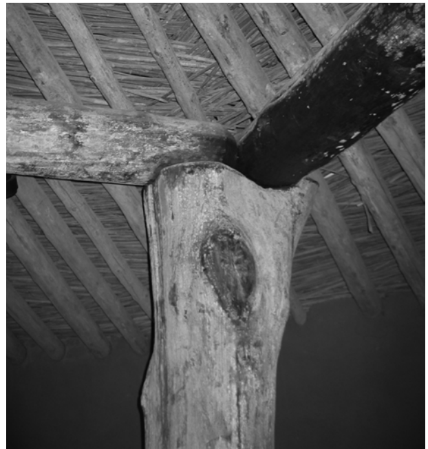
FIGURE 107. View of junction of post, beams and rafters. (NPS-SERO-CR, 2004)
