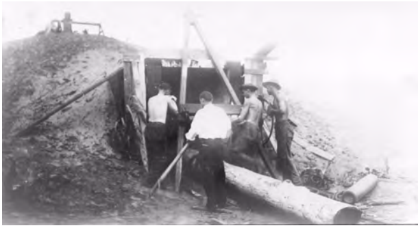
FIGURE 36. View of light derrick used to move logs into the lodge. (Swanson, OCMU Coll.)
