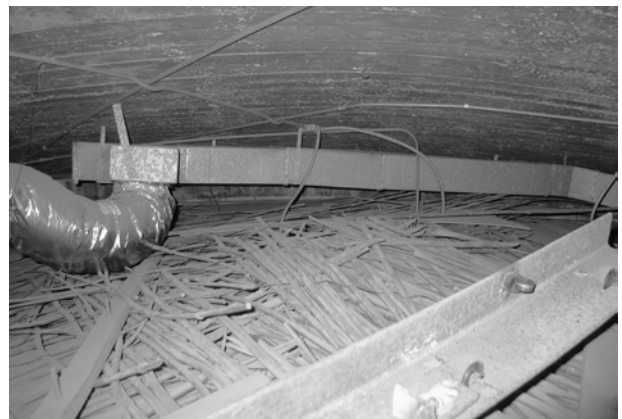
FIGURE 109. View of cane matting above main roof. Note sawn batten spiked to rafter to hold cane in place. (NPS-SERO-CR, 2004)
