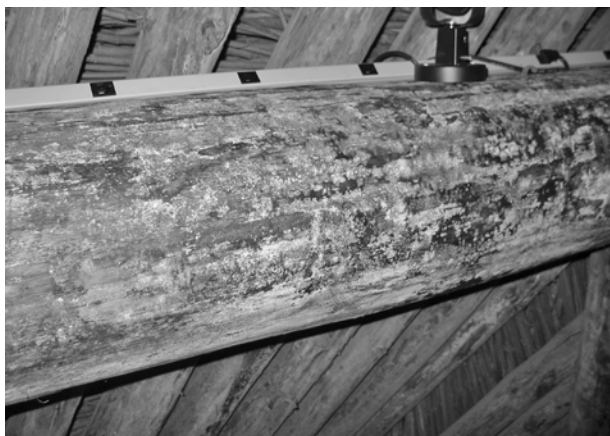
FIGURE 112. View of north beam with typical mold growth. (NPS-SERO-CR, 2004)
