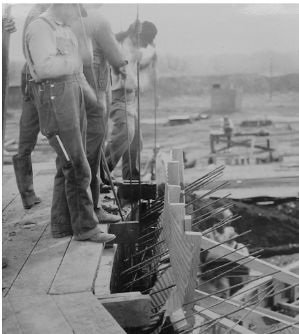
FIGURE 31. View of workmen pouring and tamping concrete wall at the Earth Lodge. (Swanson, OCMU Coll.)
