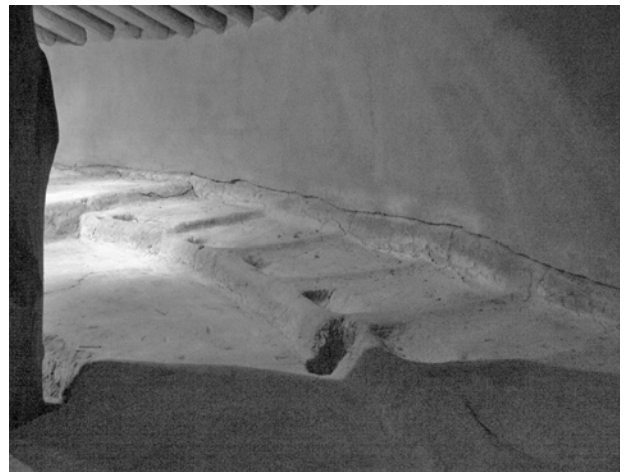
FIGURE 96. View of seats on northeast side of lodge, with highest surviving portion of encircling wall. Whitish band at base of wall is mold. (NPS-SERO-CR, 2004)
