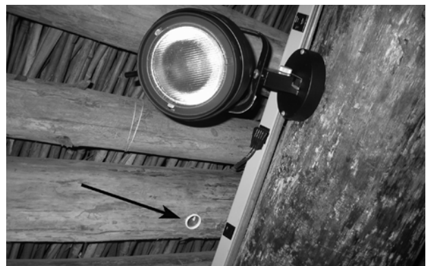
FIGURE 115. View of modern power strip and flood light. Arrow marks recessed porcelain socket for original (1937) lighting system. (NPS-SERO-CR, 2004)
