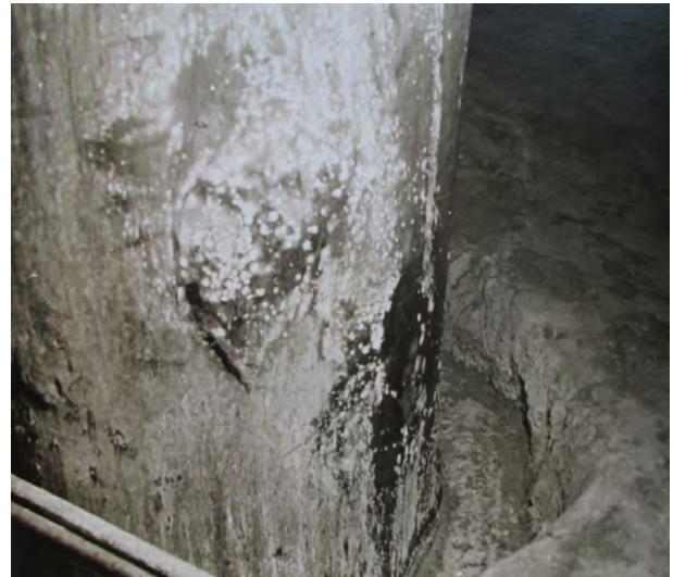
FIGURE 62. View of mold on one of interior posts, 1965. (OCMU Coll.)
