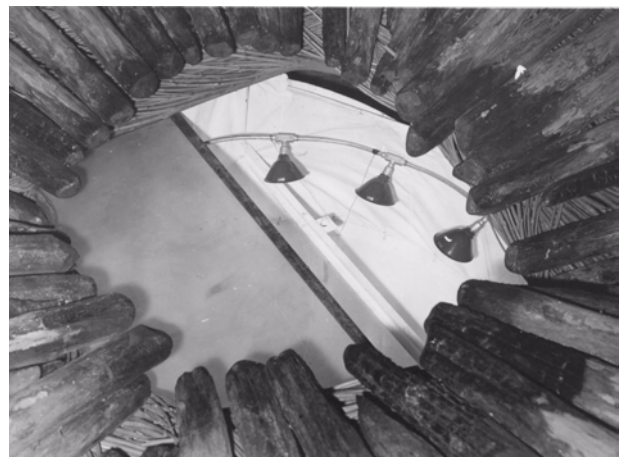
FIGURE 47. View of smoke hole with glass panel rolled partially away to expose electric lights above. (Swanson, OCMU Coll.)
