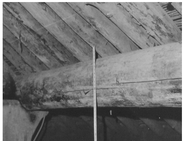
FIGURE 76. View of log which began splitting as interior of lodge dried out after installation of climate control system. . (OCMU Coll)
