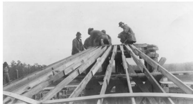
FIGURE 34. View of wooden false work for Earth Lodge roof, February 1937. (Swanson,
