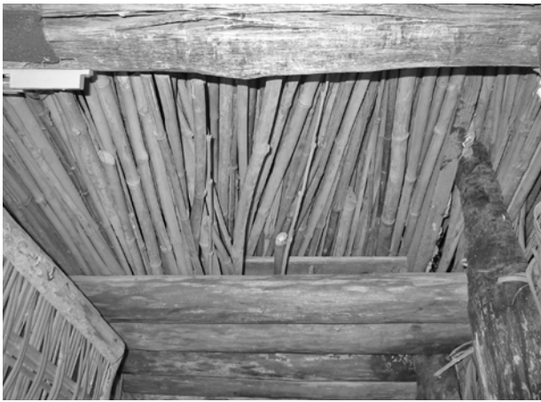
FIGURE 104. View of ceiling just inside entrance. Absence of cross logs is atypical. (NPS-SERO-CR, 2004)
