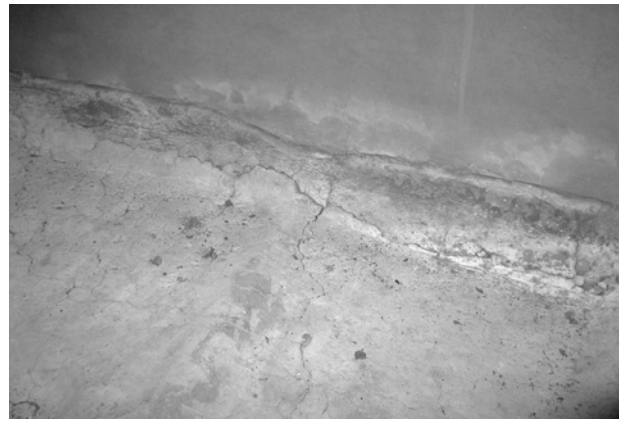
FIGURE 101. View of juncture of pre-Columbian features and reconstructed wall along northeast side. White band at base of wall appears to be mold or salts as a result of water penetration. (NPS-SERO-CR, 2004)
