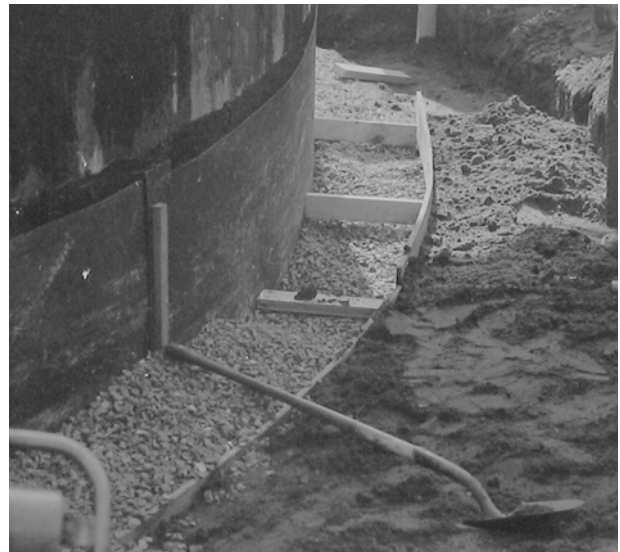
FIGURE 65. View of new French drain around perimeter of concrete shell. (OCMU Coll.)
