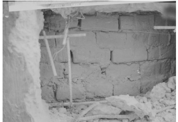
FIGURE 70. View of break in concrete shell for installation of a duct, exposing WPA-era mud brick. (OCMU Coll.)
