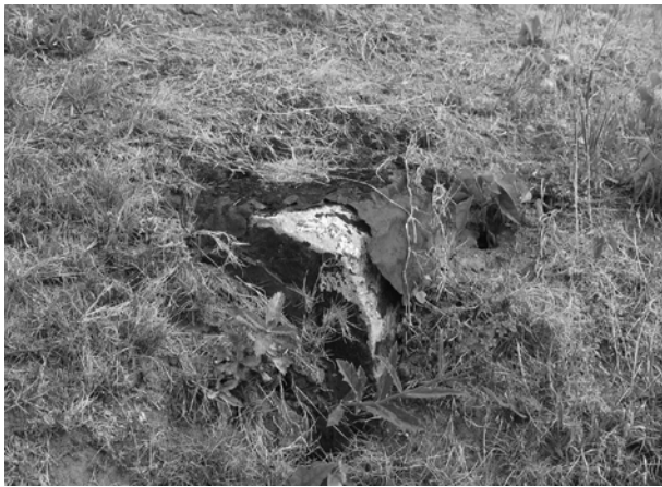
FIGURE 90. View of exposed corner of concrete shell for passageway, showing rusting corrugated metal that apparently covers the roof. (NPS-SERO-CR, 2004)
