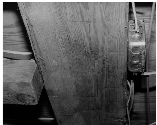
Figure 27. Typical hewn sill. (T. Jones, 1996)
