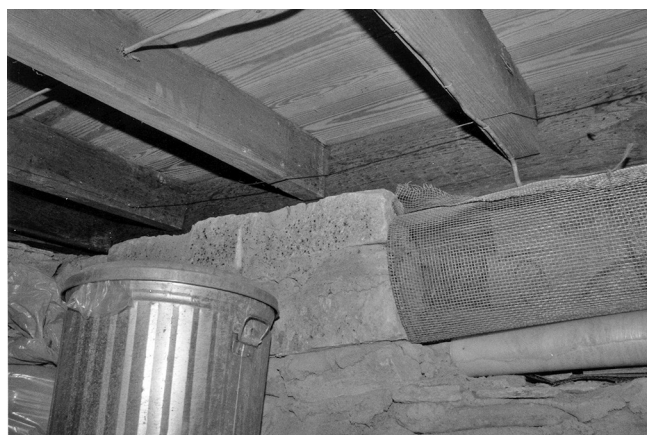
Figure 33. Cellar, looking to the southwest under Room 102, showing typical sawn joists and hewn sill.
