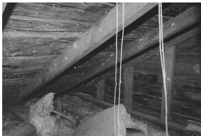
Figure 34. Attic over Room 104, looking southeast showing typical sawn rafters, studs, and decking. (T. Jones, 1996)
